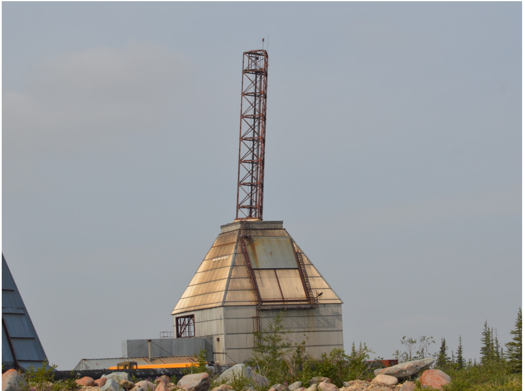
Rocket launch building
